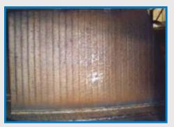
We use special linings, padding welds or anti-wear spraying which significantly elongate lifetime of fan parts. Furthermore such materials are suitable for temperature up to 600°C what allows to use these fans in a wide variety of applications.
